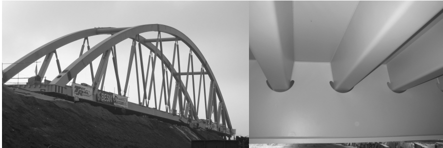
Fig. 4. Bridge over the Albert Channel before installation - Photograph of orthotropic deck of the Albert Channel Bridge, showing a crossbeam, trapezoidal longitudinal stiffeners and the cope holes
